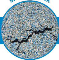
SPIDER CRACK
